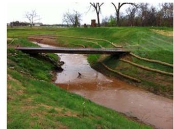
Cow creek had begun to severely erode the streambank, resulting in loss of land and increased sedimentation in the stream. This led to poor water quality and threatened buildings and utilities at the Botanic Garden. Several OSU departments and government agencies came together to develop a plan to restore the stream to a more natural state, while providing education and research opportunities.
